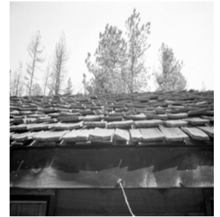
Shake shingles are still dangerous, but the cost of replacing discourages many landowners.
