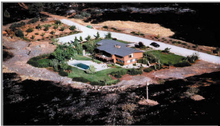
This home survived by implementing a fuel break around the yard. This fuel break forced the fire to go around due to the unavailability of fuel.
